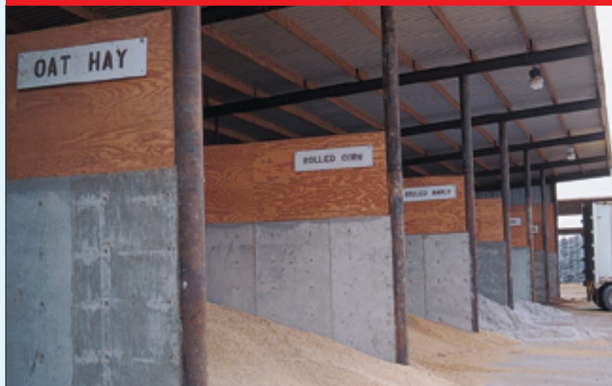
COMMODITY SHEDS with paved aprons and ample overhang make it easier to control shrink.
